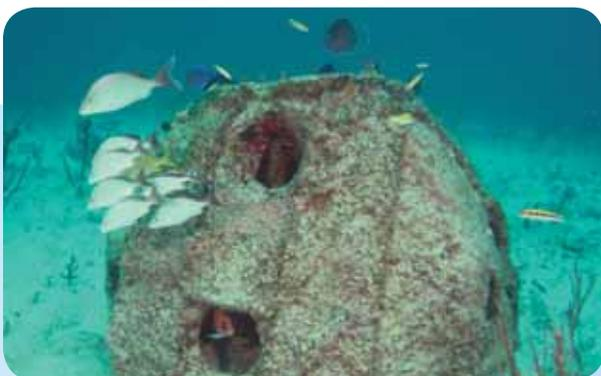
Figure 3. Substrate module with artificial invertebrate enhancing substrate pad treatment applied to the exterior.
